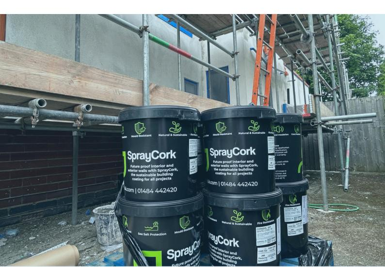
In addition, and more importantly, the natural thermal performance of the cork in CorkSol can reduce heat loss by up to 30%. The coatings are seven or eight times more insulating than traditional lime or sand renders, with a total installation thickness of 6 - 8mm. In this case, it meant that the existing render system could be hacked off and replaced without coving the lower brickwork or moving the windows.
